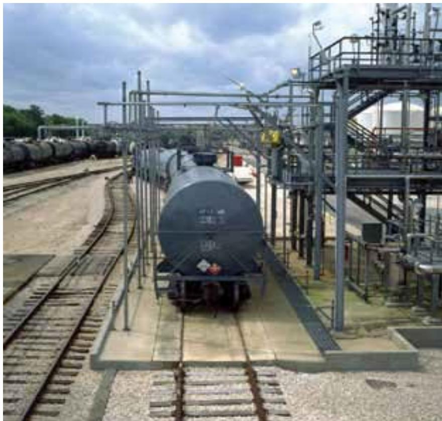
Figure 6.14 Representative layout of Ethylene Oxide unloading facilities – Pressurized transfer
