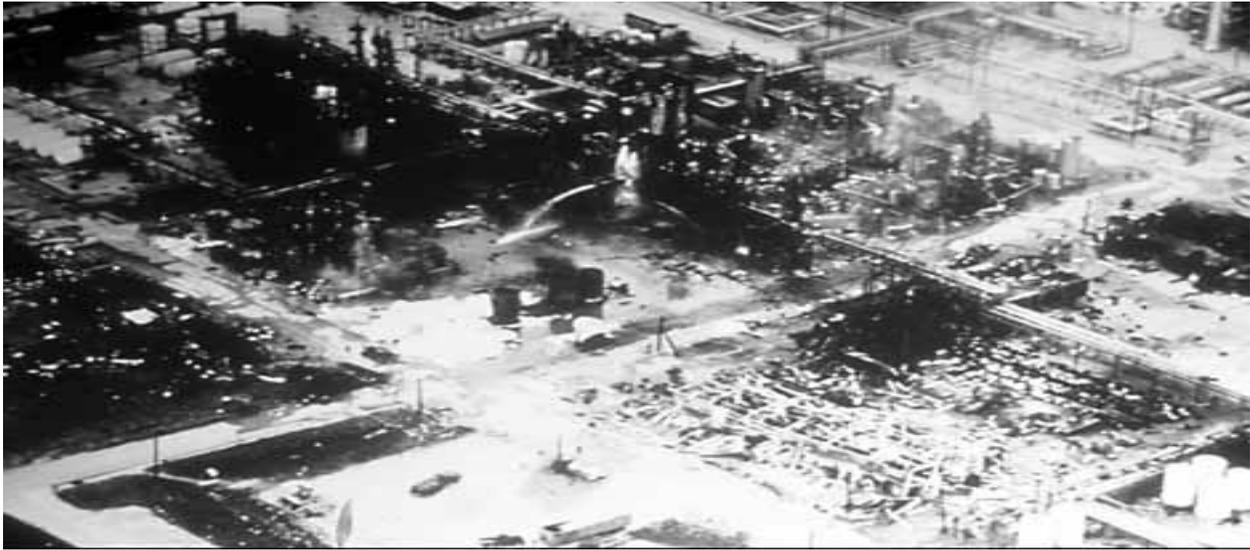
Figure 5.4 EO Tank Blown Into Process Structure 400 Feet Away
