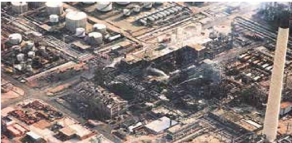
Figure 5.14 Remnants of Base of Ethylene Oxide Distillation Column after Explosion
