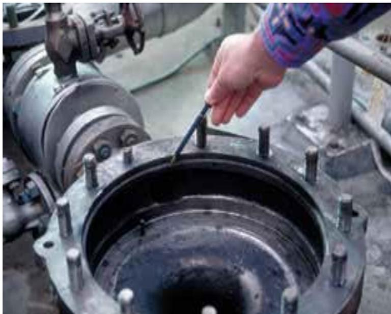
Figure 5.11 Motor Landed on Operating Ethylene Oxide Pump Discharge Line
