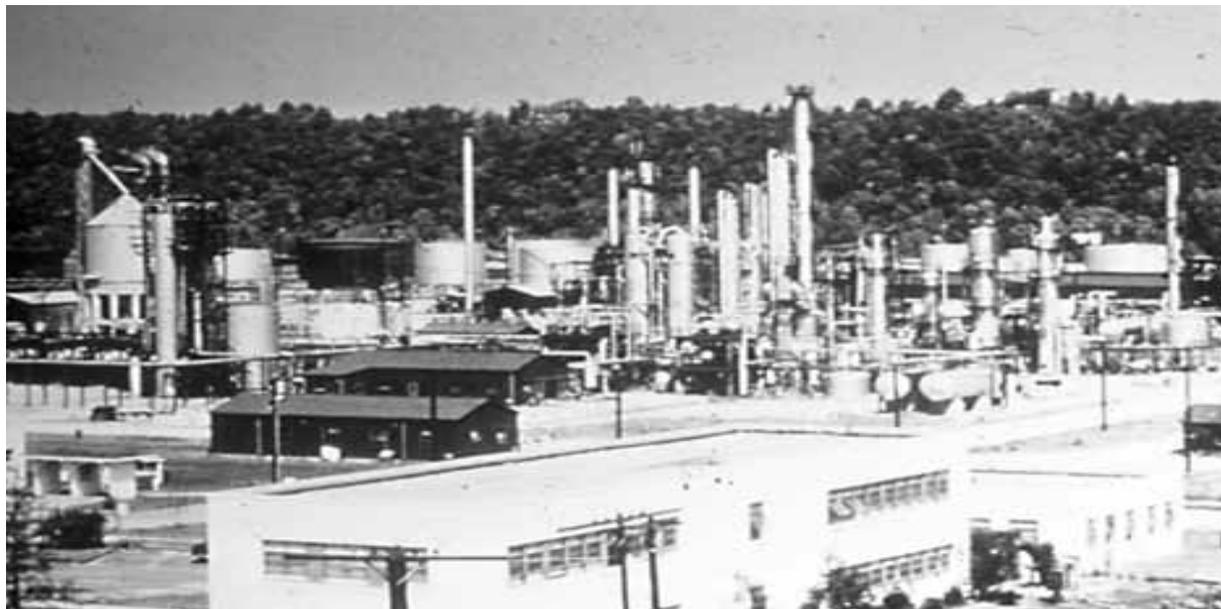
**Figure 5.2 Blast Center after Explosion – EO Vessels No Longer Visible**
